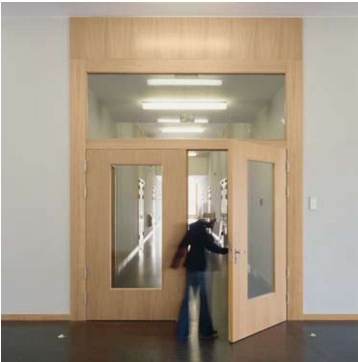
We produced this T90 door, 3.20 m wide by 3.60 m high, for the Oberstufen Zentrum (School Centre) in Berlin.
