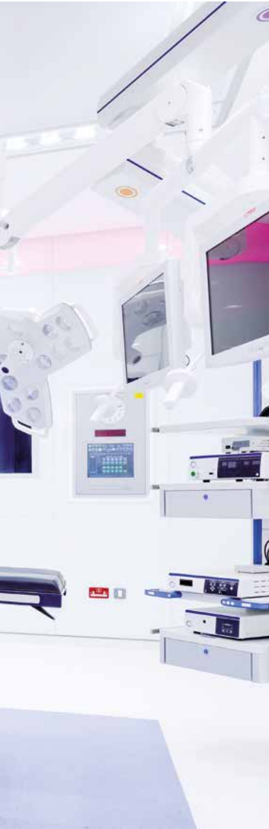
Operating theatre ceilings with low-turbulence laminar airflow system / Zu-/Umluftdecken zur Versorgung der Operationssäle
